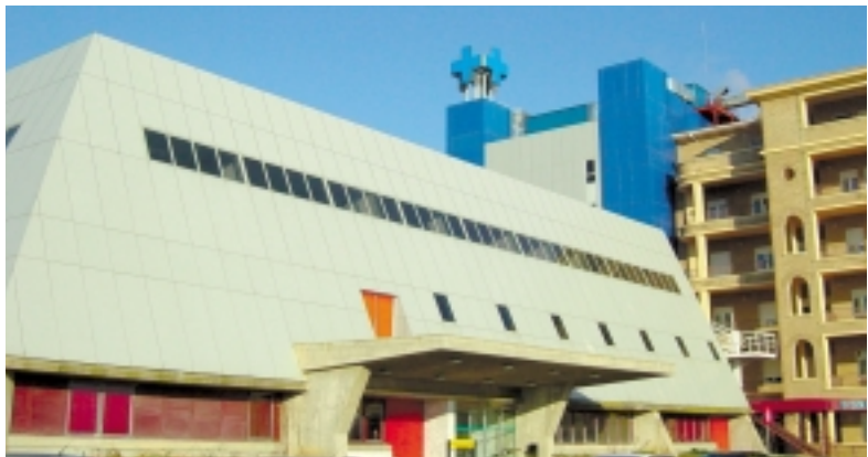
Hospital Royo Villanova
